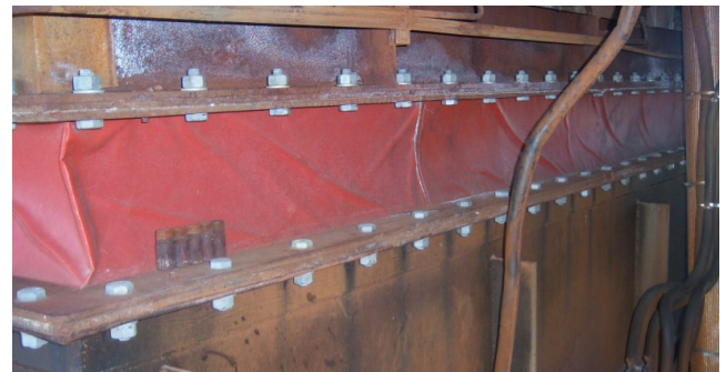
NON Metallic, NON Insulated Expansion Joint
