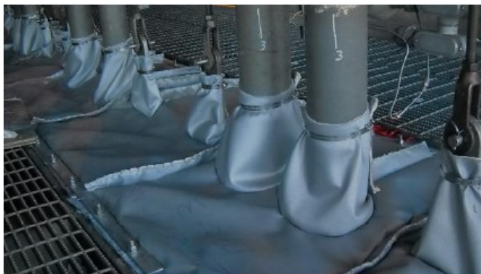
Deck Seals installed on a SWEC furnace
